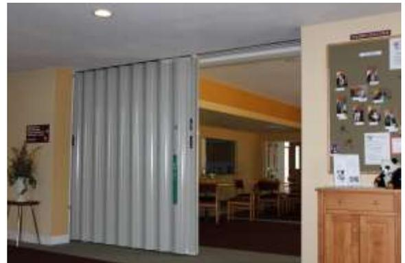
The fire door between the Lobby and Gathering Place will close blocking travel between the two areas on the main level of the building. The fire door CLOSSES IN LESS THAN 15 SECONDS.
